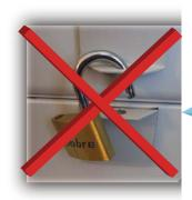
Notice how the plates are positioned too far apart for the lock to close.
